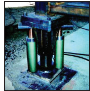
Contractors called on the brute force of Simplex R5513 cylinders to lift and position highway ramps in San Diego. G6 provided the power and control in this rough outdoor application.
